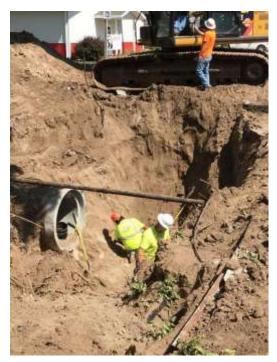
The project in mind was to replace and expand the existing storm sewer system. Instead of the 24" pipe, there would be a 36" pipe that would increase the capacity from 9 cubic feet per second
